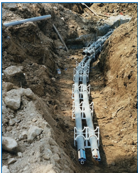
Pulled through existing conduits
